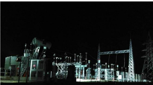
110kV Switchyard for 20MW Ground Mounted Solar Plant Ramdurga, Karnataka
